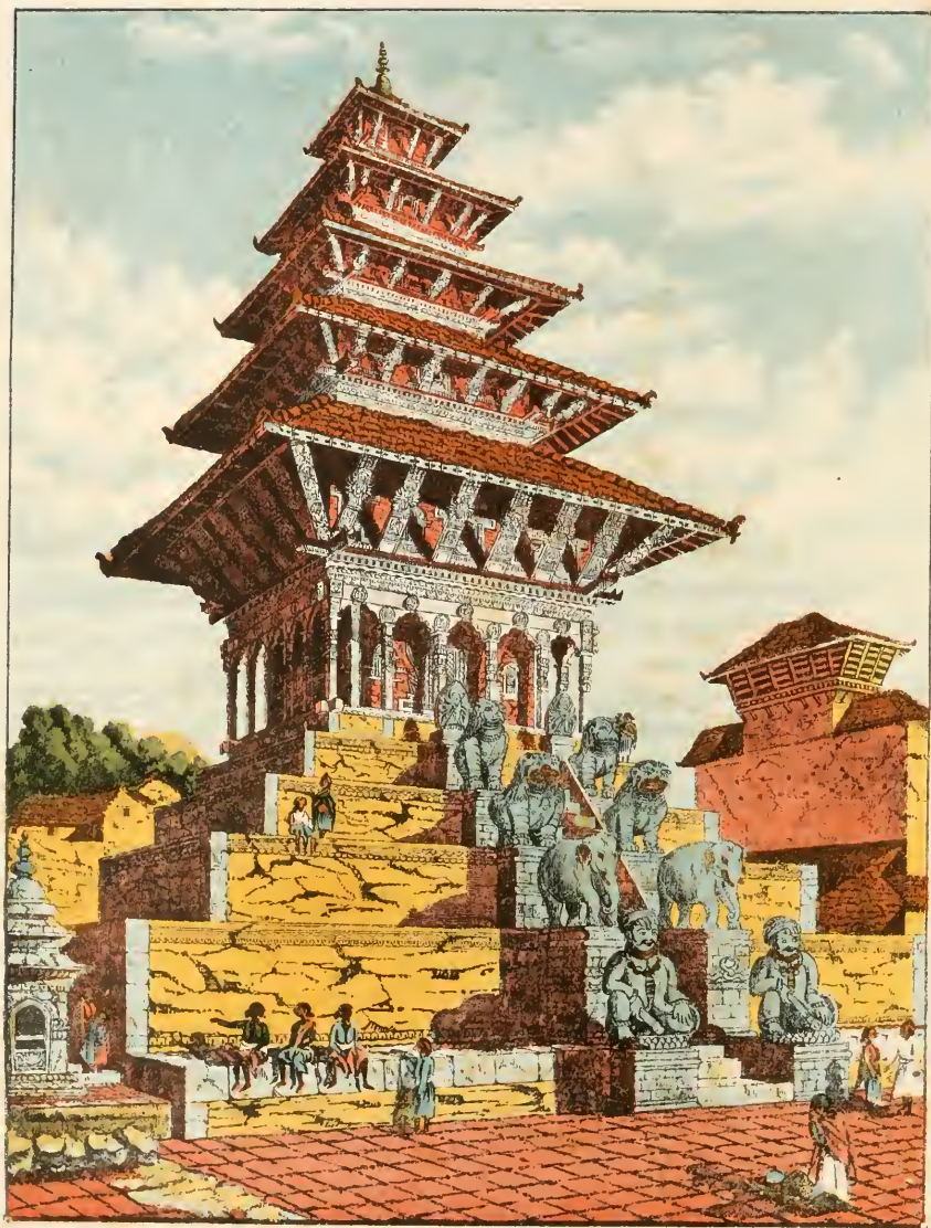
TEMPLE OF DEVI BHAGWANI, BHATGAON. Built, A.D. 1703.
