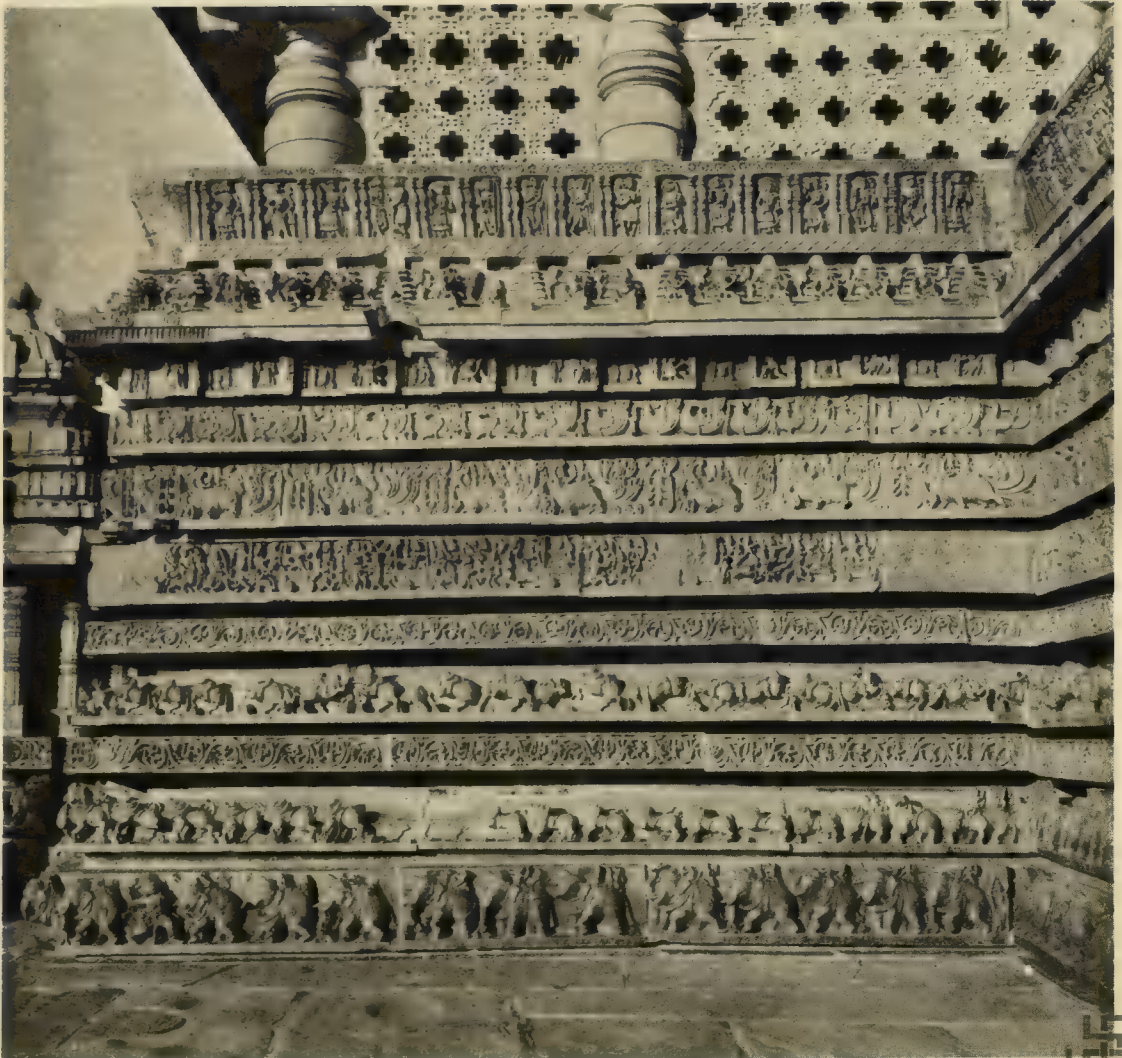
Fig. 7. A section of the outer wall, Hoysaḷēśvara temple. 1967.
