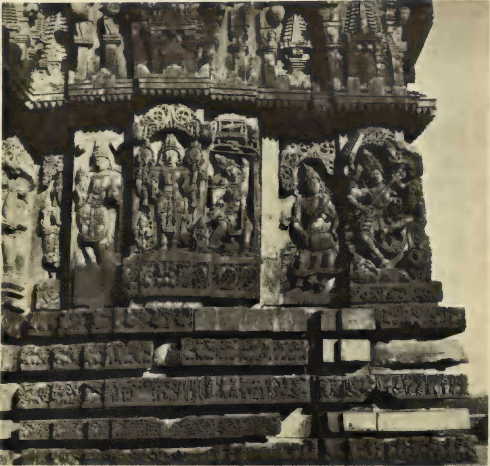
Fig. 14. Restored outer wall of the Kēdārēśvara temple with missing basement friezes. 1969.
