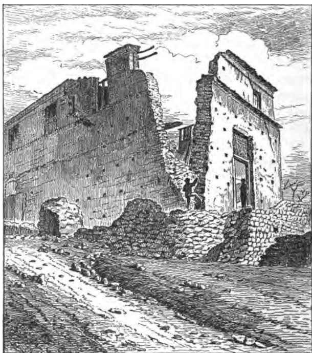
FIG. 19.—The Cathedral, Paterno (Mallet). Neapolitan Earthquake of 1857.
