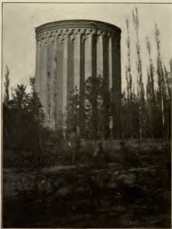
TOWER AMONG THE RUINS OF REI, AFTER RESTORATION
