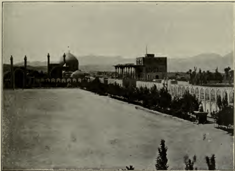
THE MEIDAN OF ISFAHAN The Royal Mosque and the Porch of the Palace
