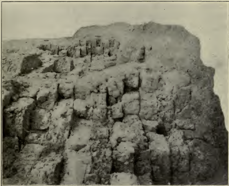
CRUMBLING WALLS OF REI
