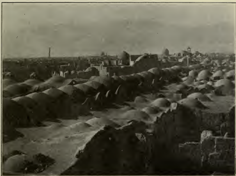
DOMED ROOFS OF KASHAN
