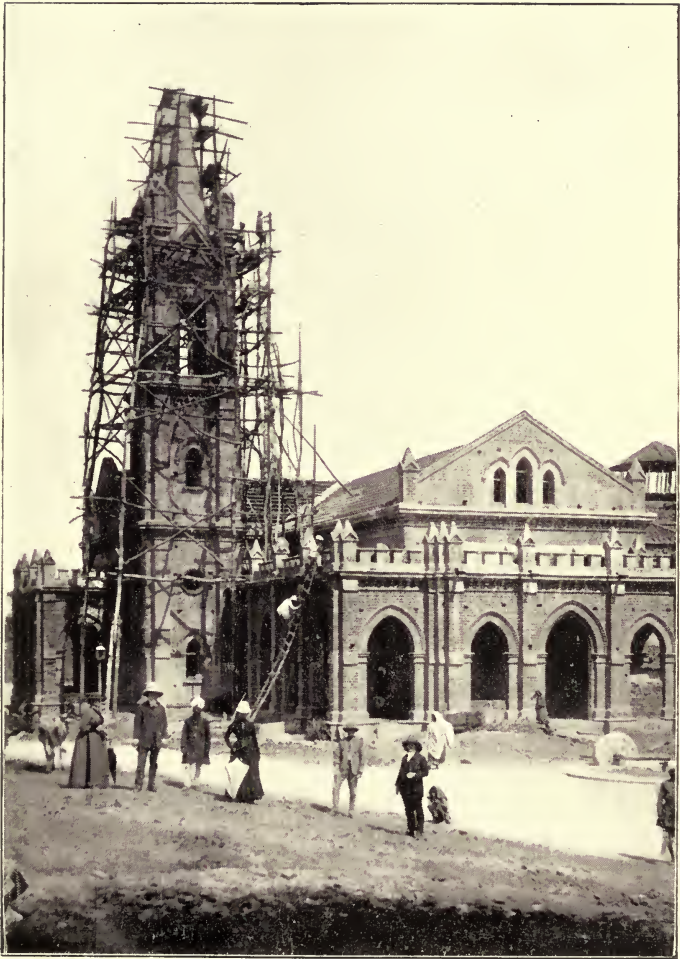
CHURCH IN COURSE OF ERECTION.
