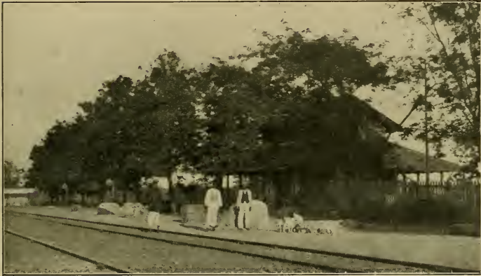
RAILROAD STATION AT NAVAPUR.
