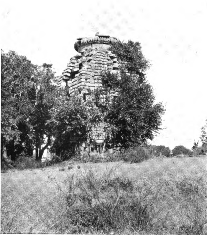
TOWER IN PROCESS OF DESTRUCTION BY TREES, BHUVANESWARA.
