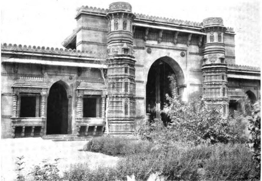
QUEEN'S MOSQUE IN MIRZAPUR, AHMEDABAD.
