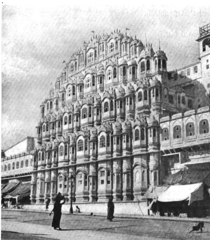
BUILDING AT JEYPORE.
