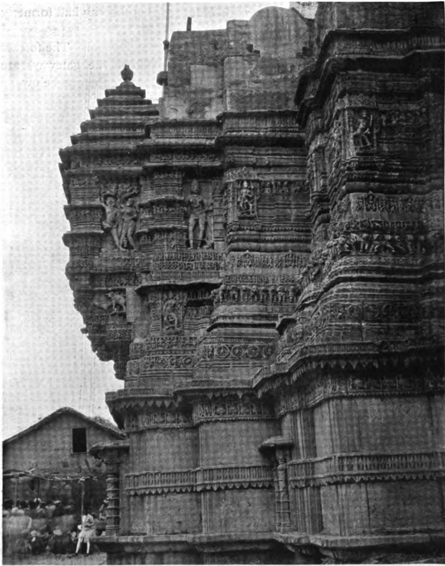
KALIKA MAHTA TEMPLE, OUTSIDE HIRA GATE, DABHOI.
